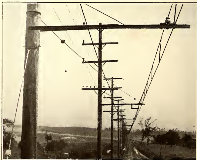
VIEWS ON SAN BERNARDINO LINE OF PACIFIC ELECTRIC RAILWAY SHOWING OVERHEAD CONSTRUCTION WITH STEEL CONTACT WIRE
